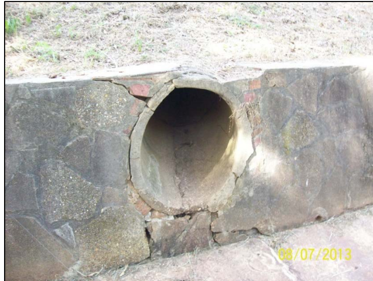
Photo 4 – South Subsystem A 24” RCP outfall downstream of 48” pipe
