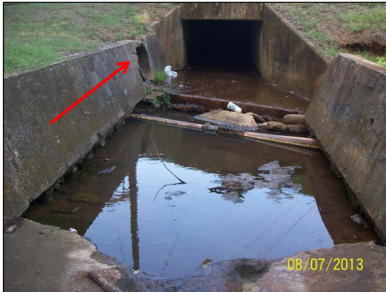
Photo 2 – 24" RCP outfall of North Subsystem A
