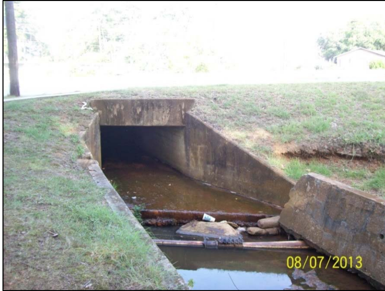
Photo 1 – 7'x4' RCB outfall underneath U.S. Highway 259 discharging to a concrete-lined channel
